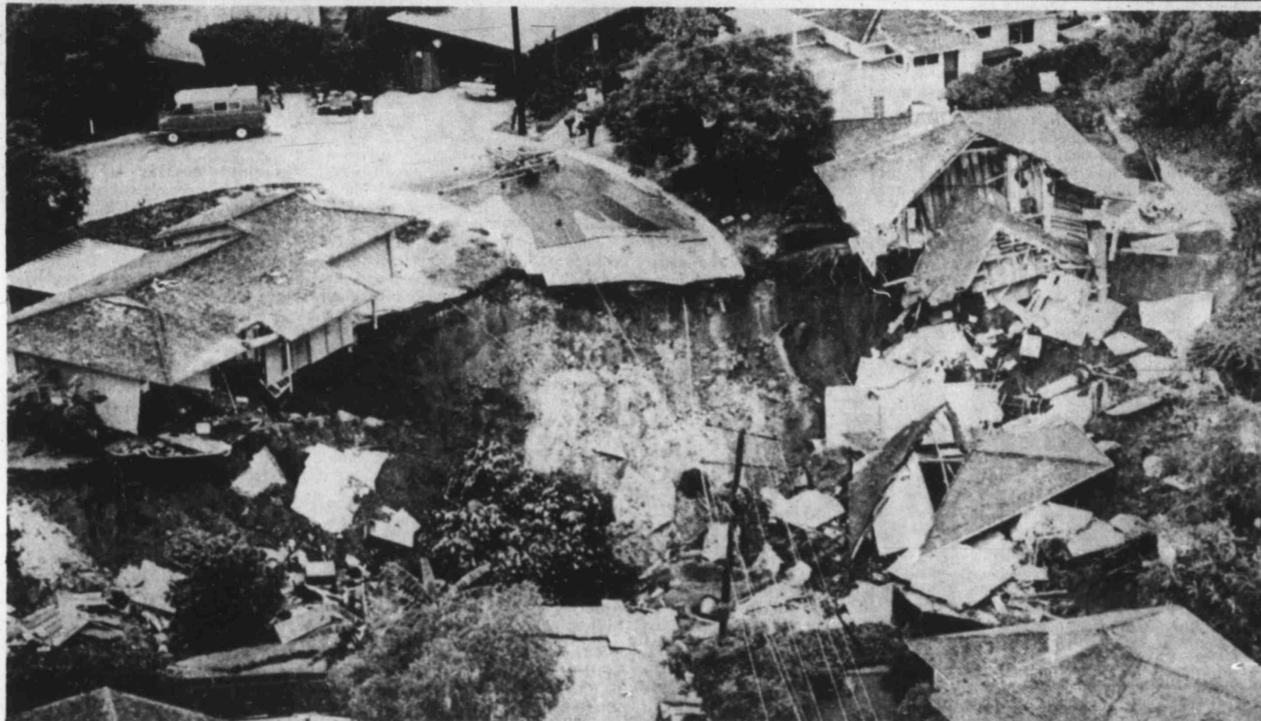
This is a section of fashionable Laguna Beach, Calif., where an early morning landslide destroyed some 20 expensive homes and damaged others. Several injuries were reported and several power poles were down and gas lines ruptured. (AP Laserphoto)
