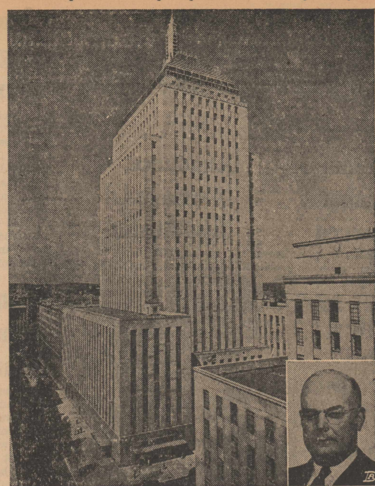
BOSTON—Tallest building on eastern seaboard between New York and Canada, John Hancock Mutual Life Insurance Company's new 26-story home office building was opened officially with Secretary of the Treasury John W. Snyder, inset, as principal speaker. This is first photo of recently completed structure minus scaffolding.
