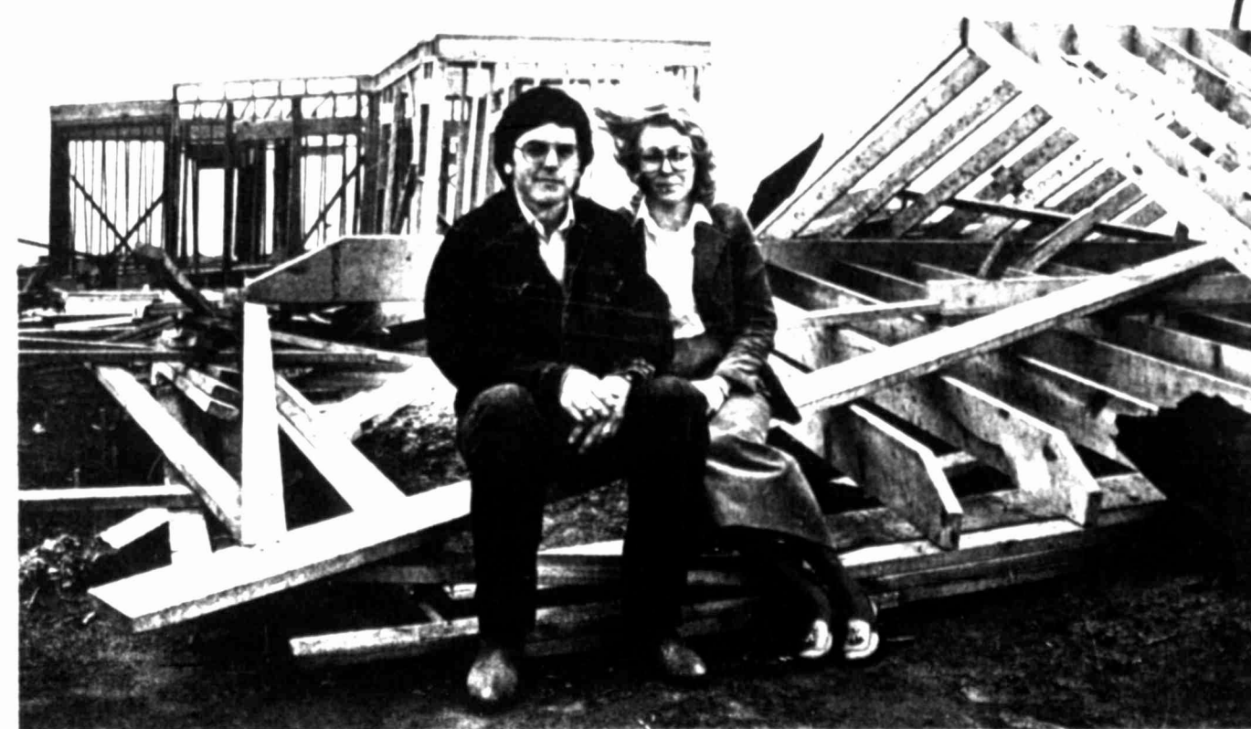
Mr. and Mrs. Bill Thomason, contractors for the 62 home Lafayette Place subdivision on North A Street near Wadley Avenue, sit Friday afternoon on the contorted framework of what was to be their new two-story home. According to the Thomasons and several other persons on the scene at the time,
