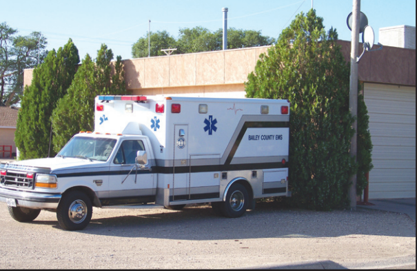
Bailey County EMS building
