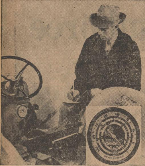
FORD TRACTORS now coming off the assembly lines at the Ford Highland Park, Michigan, Plant are equipped with the new Proof-Meter, an instrument which "takes the guesswork out of tractor operation." Actually five instruments in one, the Proof-Meter shows engine speed, tractor speed, power take-off speed, belt pulley speed and total hours
