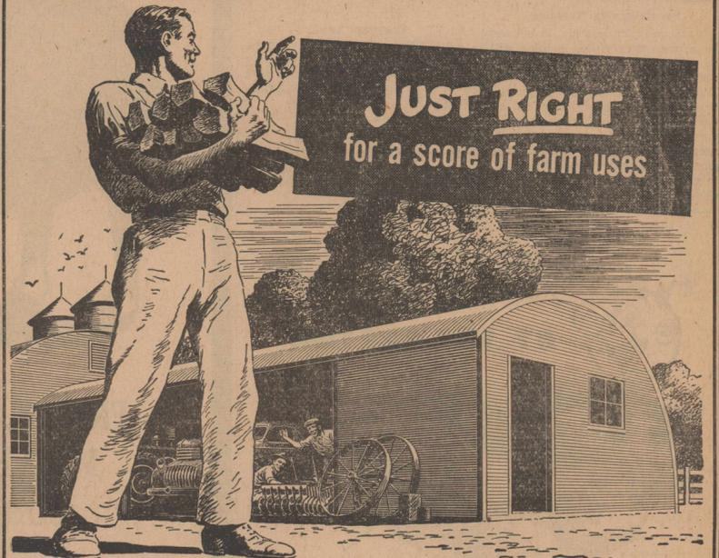
Here is one of the countless variations of the "Quonset 24." Three sections are used as an implement shed; the fourth section, enclosed and fitted with walk-door and window in side panel, makes an ideal workshop.
