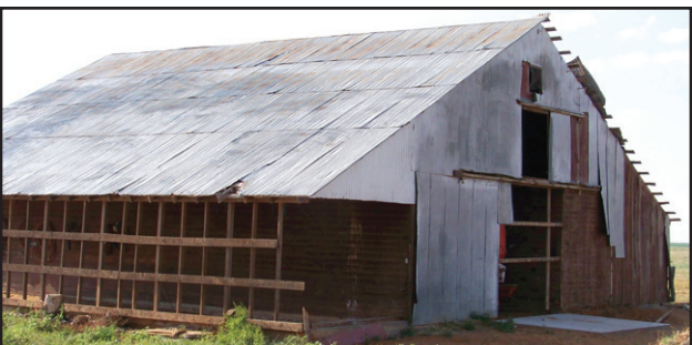
The old metal barn stands ready for repair.
