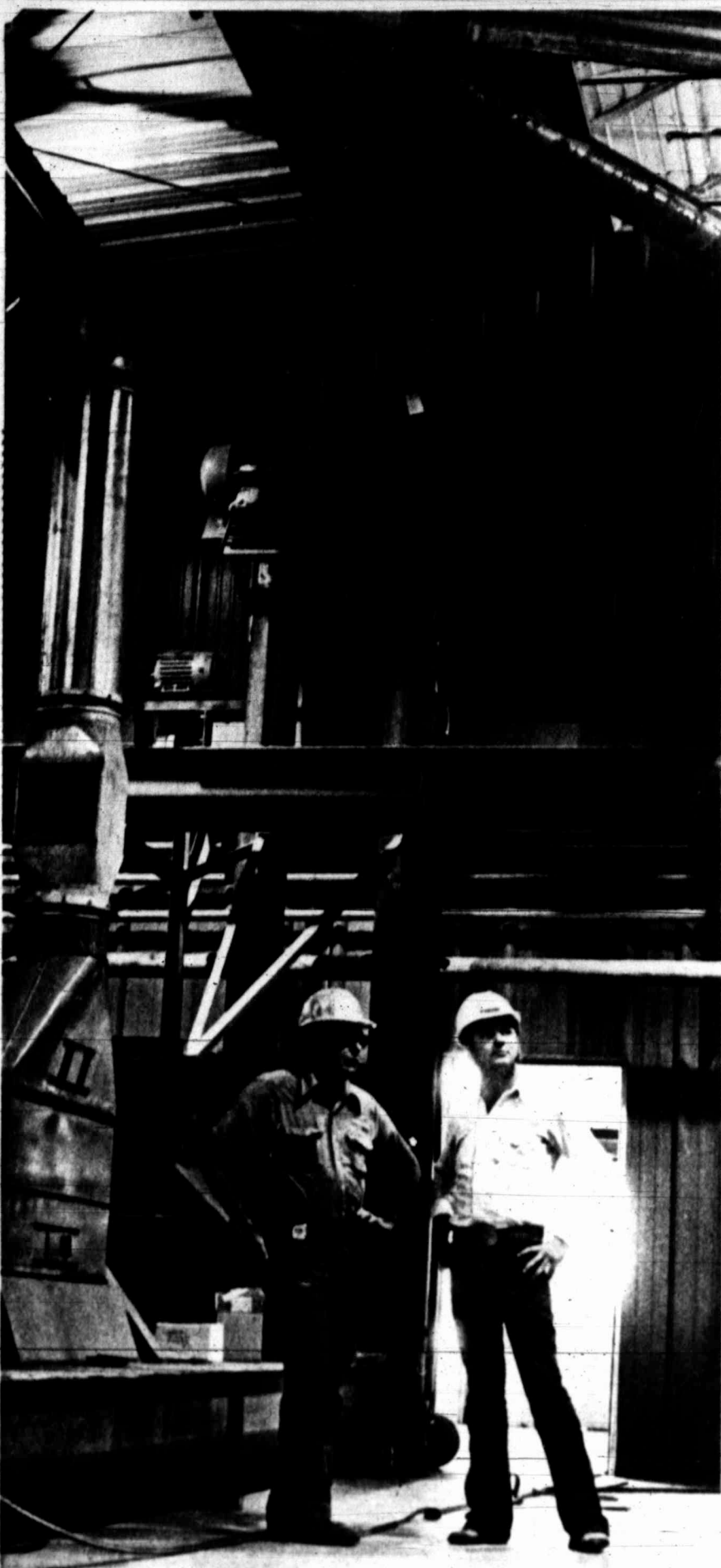
Robert Pearson, left, of Lamesa, superintendent of the Lamesa Cotton Oil Mill, and construction foreman Rick Northcott of Lubbock look over new equipment at the cottonseed oil mill. The original mill was built in 1937-38. (Staff Photo by Ed Todd)
