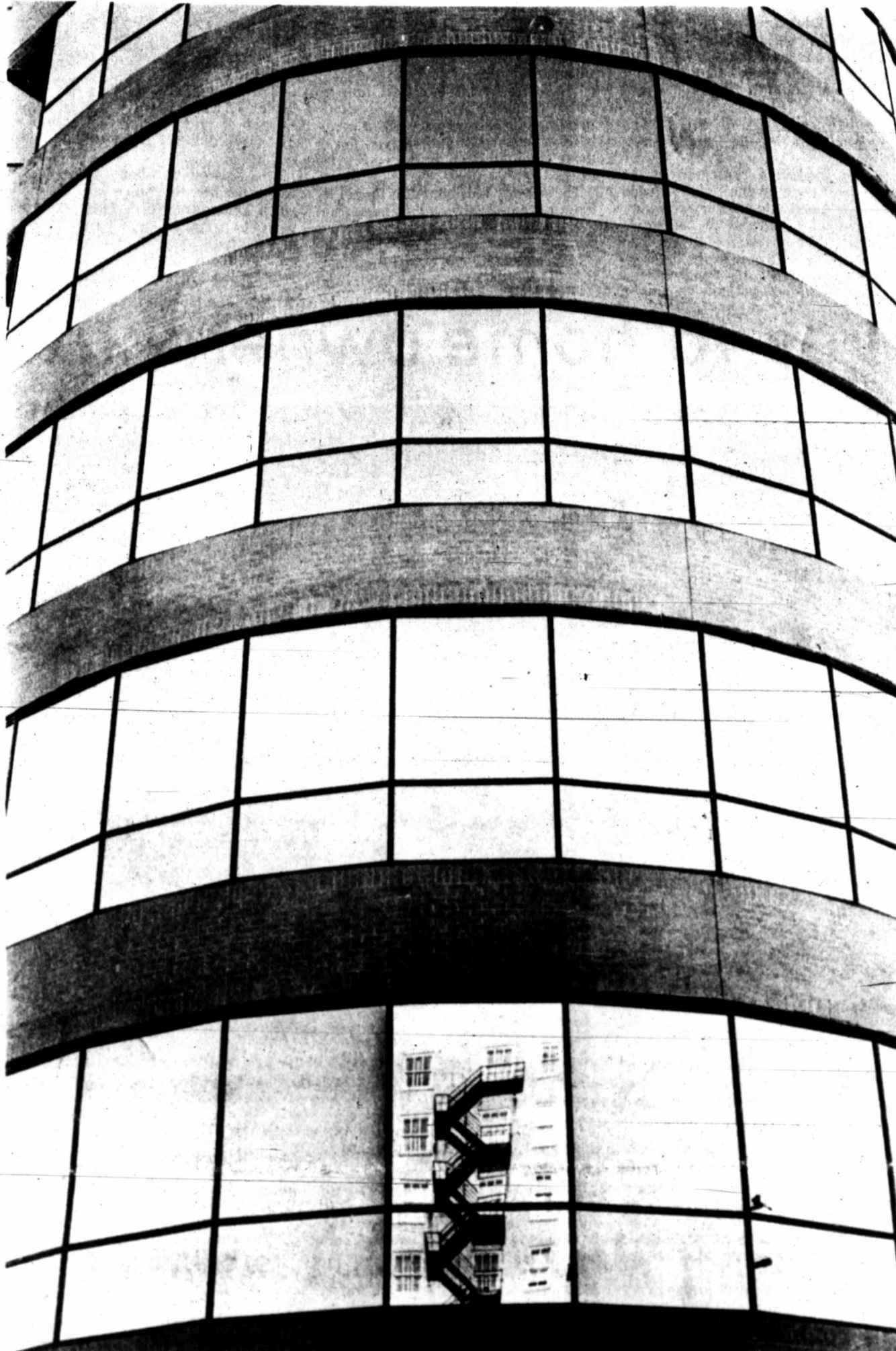
It will be a long trip to the top of the 15-story Gibraltar Savings Building at Texas Avenue and Loraine Street, but the little stairs on the southwest
