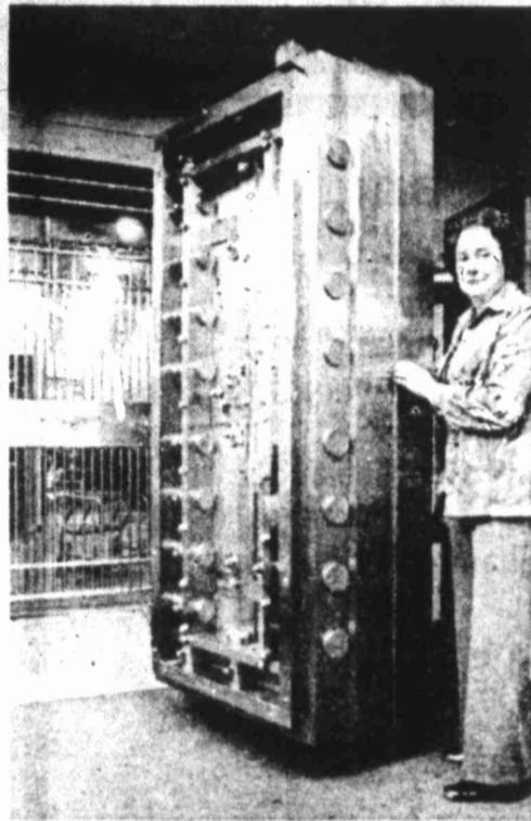
Banks store money in vaults with doors that can be 2 feet thick. The doors have combination locks that will not open until a special time.
