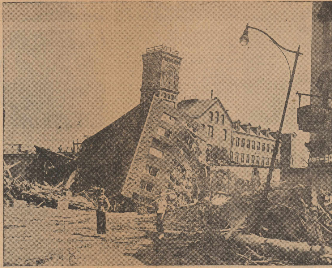
CRUSHED AND BROKEN, this 16-family apartment house in Waterbury, Conn., was left high and dry after the rampaging Naugatuck River receded August 21. This was a sample of devastation in the flood which, according to the Red Cross, destroyed 1,326 houses and badly damaged 4,808. (Wide World Photo)
