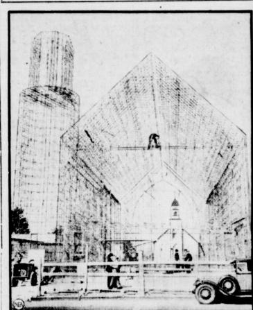
of small rods interwoven to form a network of steel welded into a single unit, St. Augustin's Catholic church, shown above, in
