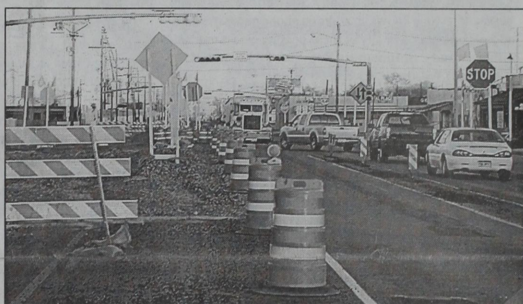
Road construction at the intersection of Highway 214 and US 84
