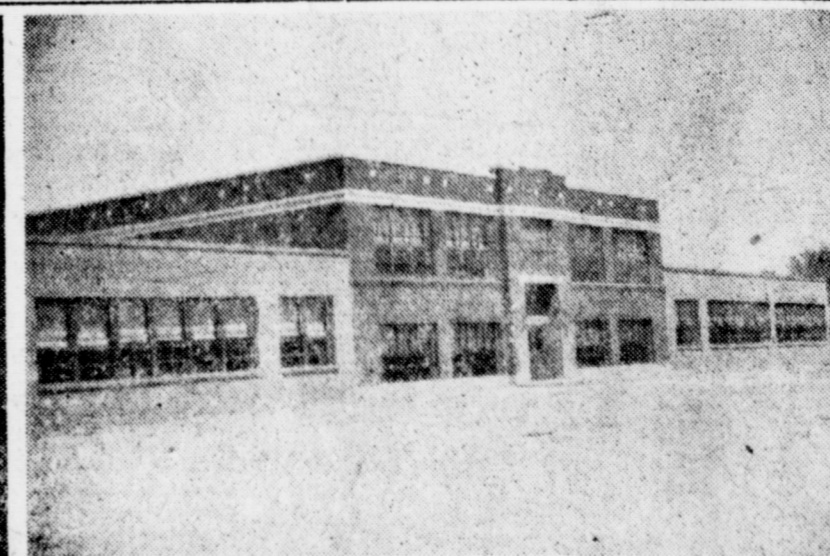
ELEMENTARY SCHOOL — The lower grades of the Muleshoe school district will attend classes in this building. It is recently remodeled and is in very good condition. Before the new high school was completed, it was the best plant in the school system. Photos by members of The Journal Staff.
