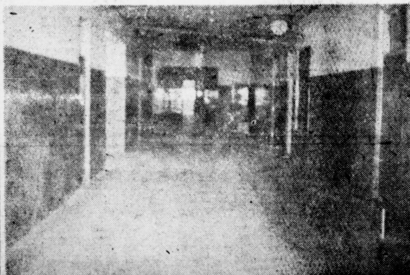
BEAUTIFUL CORRIDOR — This is a view of the hall connecting the auditorium with library in the new high school. At the far end is the library entrance. All floors and the wall almost to the top of the doors are made of green terrazzo and the doors are made of highly polished oak veneer. Classrooms are located on both sides of the hall. Entrance to the superintendent's office is located under the clock.
