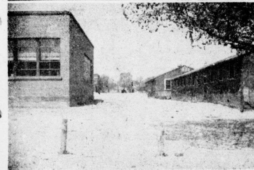
CAMPUS EYESORE — Several unsightly old barracks buildings on the north side of the campus have been used for the classrooms and other school needs. The new high school building will eliminate most of them. Note tar-paper covering coming off the building at right. The others are in like condition.
