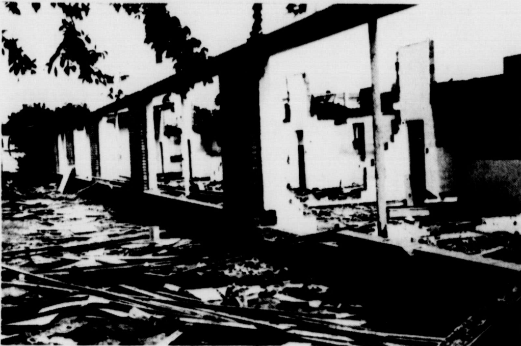
INTERMEDIATE SCHOOL BEING TORN DOWN
