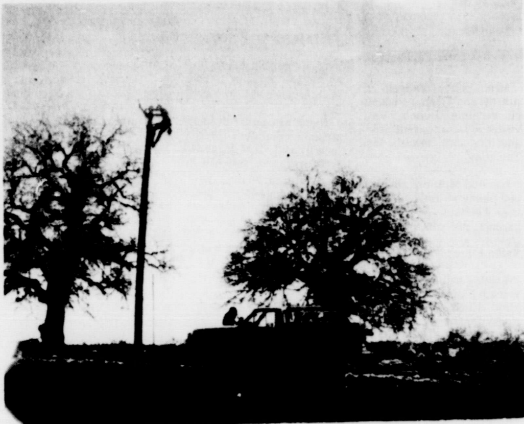
FIXING LINES-- West Texas Utility workers put in over 30 hours this last holiday weekend to fix downed power lines across Cisco. The lines fell due to the heavy ice on them from the ice storm that came across the big country on Saturday morning. Homes on the Lake Bernie road were without electricity for about five hours and some homes south of town in the country were without electricity for a short time according to a report from the WTU office. (Staff Photo)
