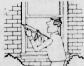
Caulk around doors and windows
