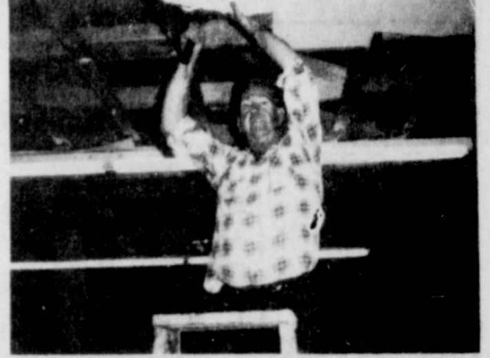
Lloyd Swindle removes ceiling material from City Library ceiling.
