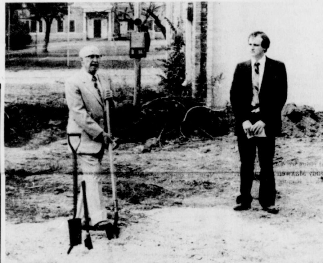
CHAIRMAN Standlee McCracken of the building committee was about to turn the first shovel of dirt to begin work on a new $100,000 wing for the First Christian Church building when the above picture was made at Sunday's ground breaking ceremonies. The Rev. Milo Steffen, right, presided at the event.—Staff Photo.
