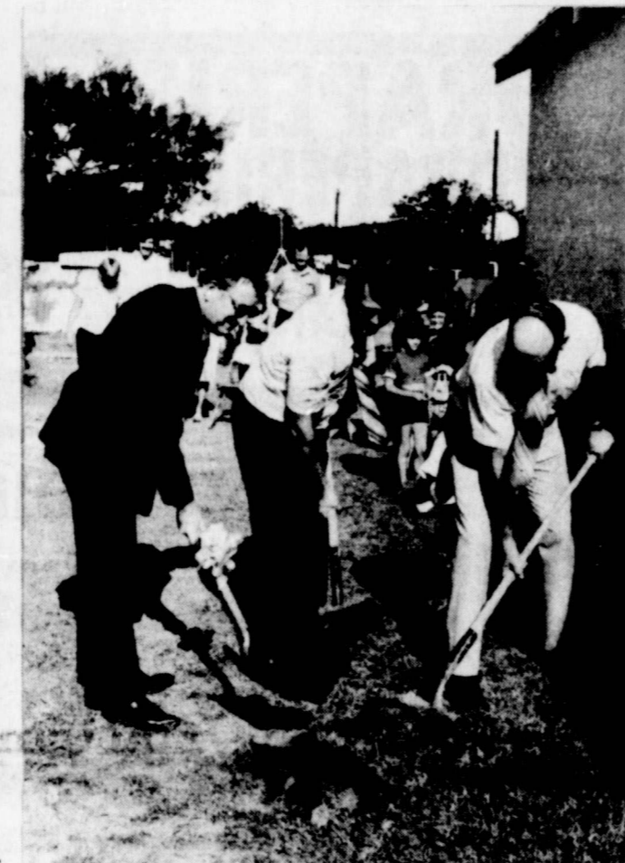
GROUND BREAKING ceremonies were held last Sunday at Calvary Baptist Church in Cisco. Shown in the above photo are (left to right): Rev. Cecil Deadman, pastor of East Cisco Baptist Church; Rev. Ronnie Shackelford, pastor of Calvary Baptist Church; and Wayne Webb.
