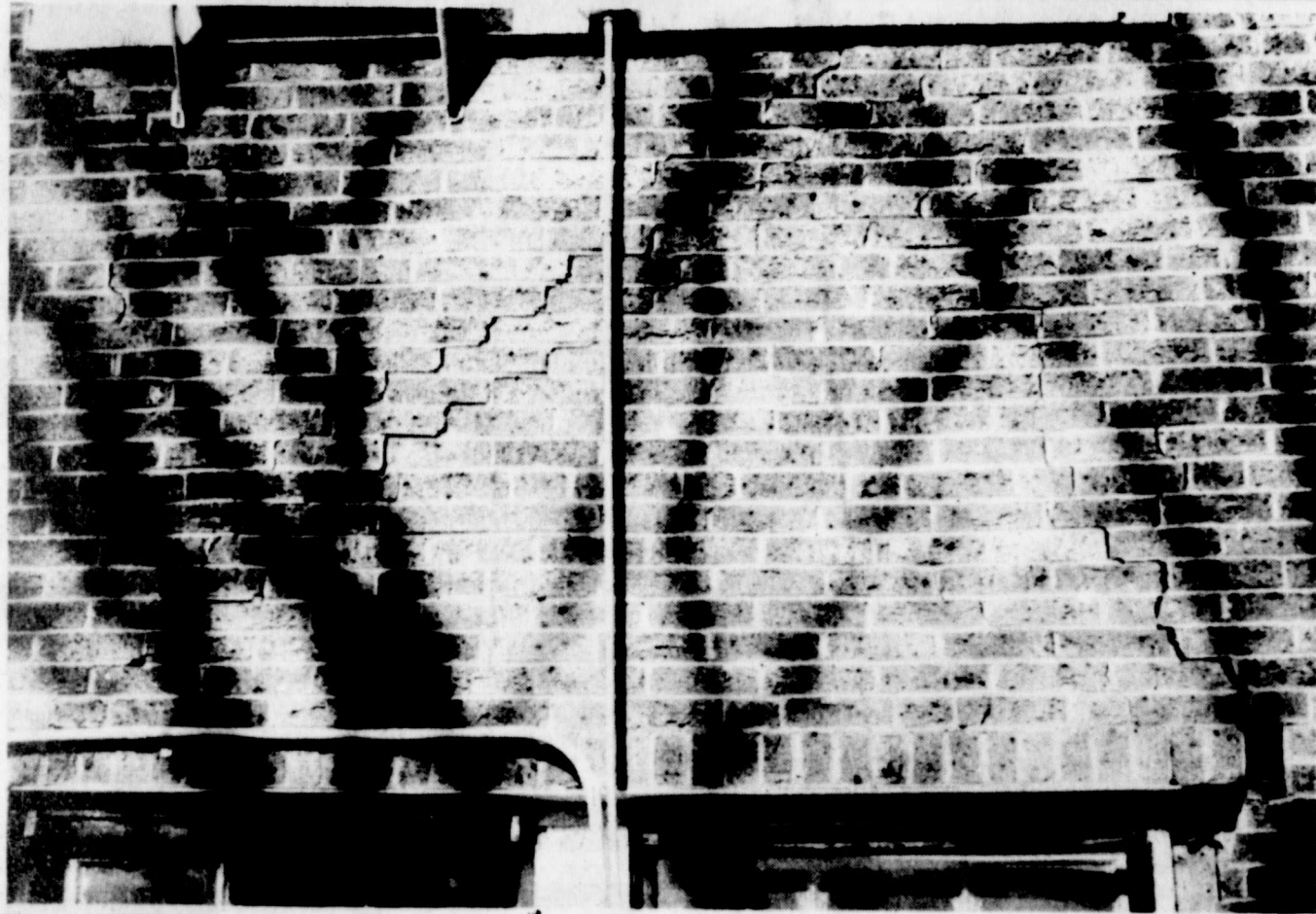
NEW CRACKS in the brick wall on the west side of City Hall showed up last weekend and City Manager Mike Moore ordered the area near the wall to be roped off due to possible danger. Mr. Moore said the ropes would stay up until competent technicians are brought in to examine the wall and determine the problems. (Staff Photo)
