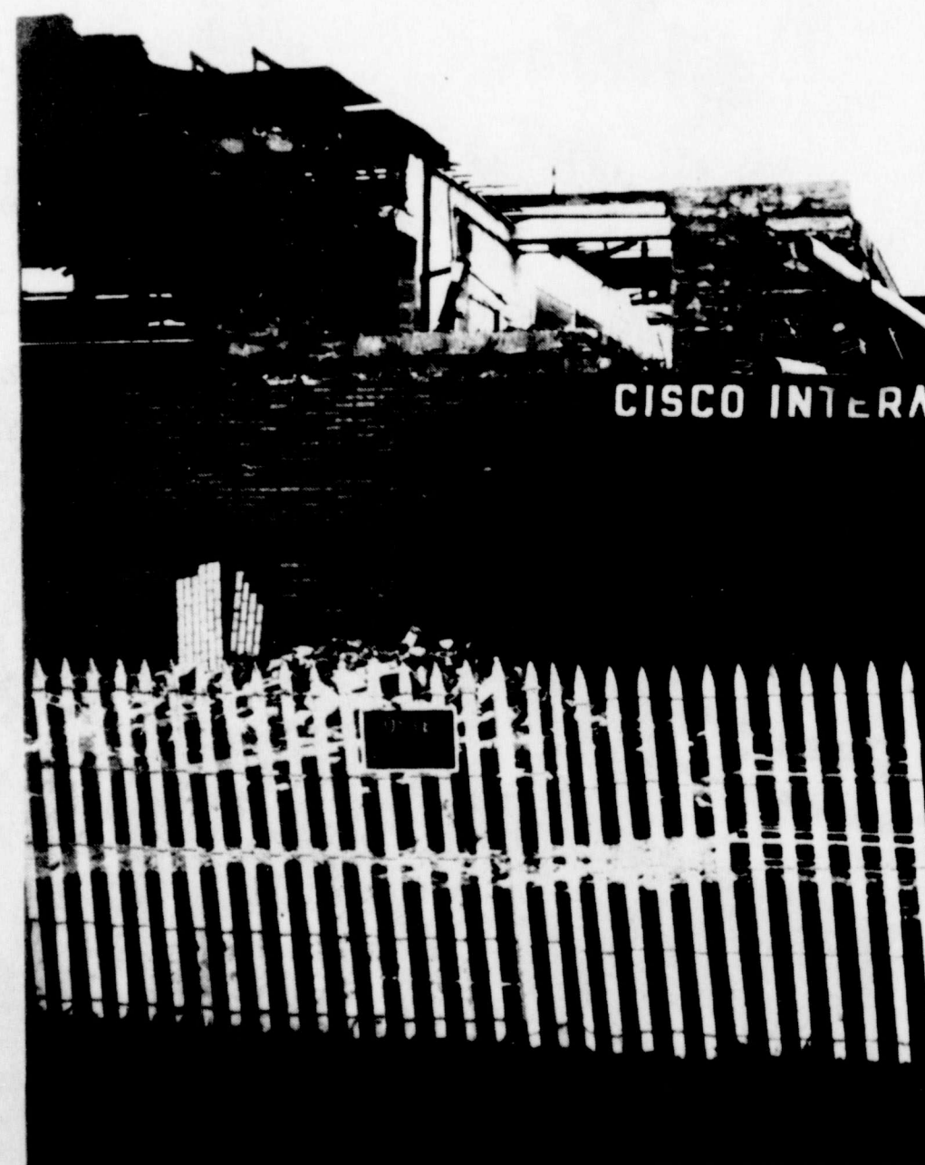
COMING DOWN-- The gymnasium at Cisco Intermediate School, damaged last year by a windstorm, was being torn down this week by Bontke Brothers Company. The demolition contract was awarded by the Cisco School Trustees last week. In the two photos above, taken Wednesday, the northeast corner of the building was being torn away from the part of the building which will be left standing. Thursday afternoon, the east walls of the gymnasium were pushed down by a bulldozer. (staff photos)
