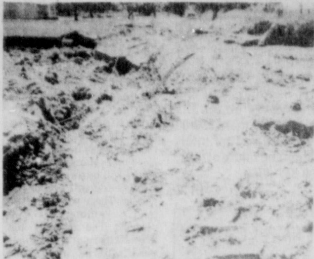
What road are we talking about here? This picture shows all that remains of a section of Rd. No. 419, near Highway 8 at Gorman. Comm. Christian reports that this road will take 960 yds. of material to rebuild.
