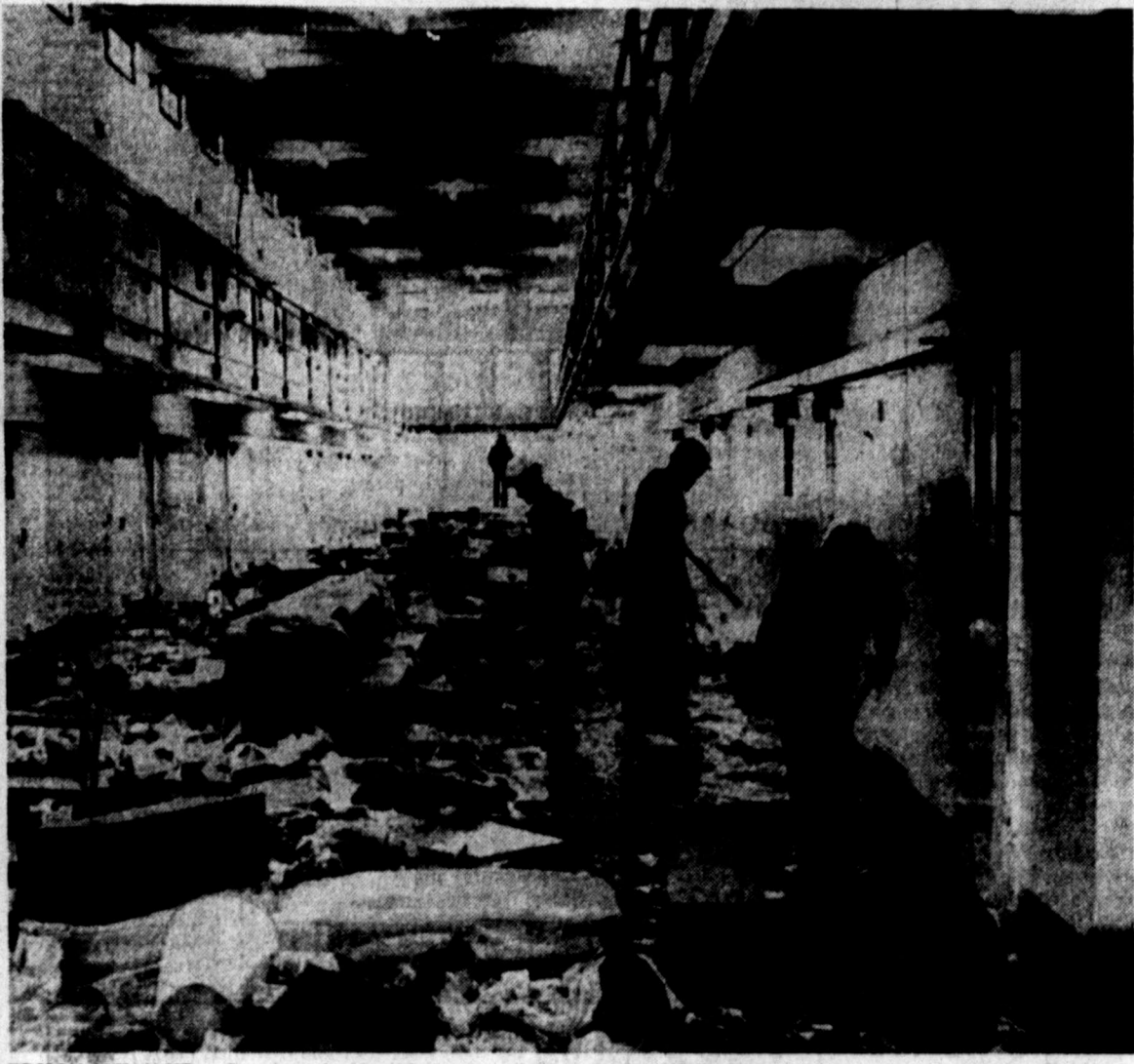
PRISON CLEAN-UP — Guards at the New Mexico State Penitentiary work to clean up cell block six at the prison Monday. Prison officials have estimated $40 million in damages done to the institution during weekend rioting by inmates. At least 35
