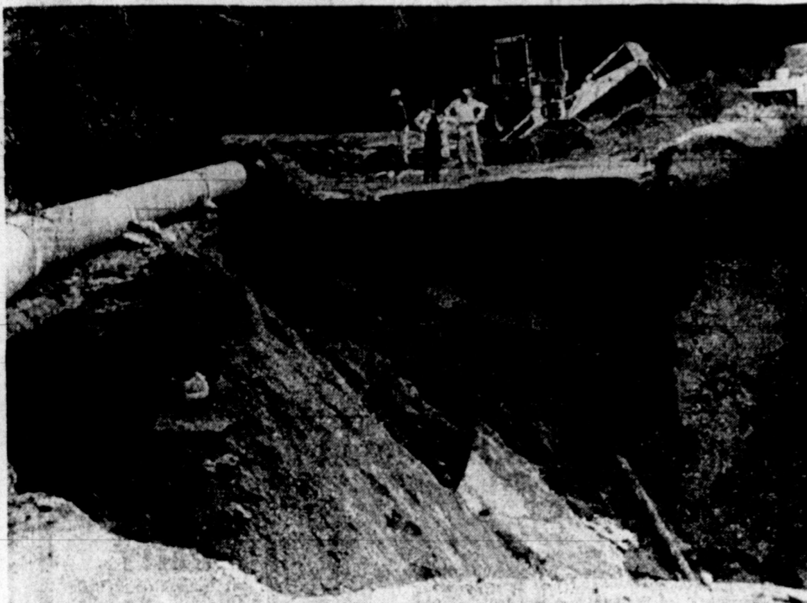
BIG POTHOLE — An unidentified couple stands near work crew at the edge of a huge hole, all that's left of a section of Nichols Canyon Road in Los Angeles after heavy rains and mudslides washed the road surface away over the weekend. On the heels of "one storm right after the other" the death toll Mon-
