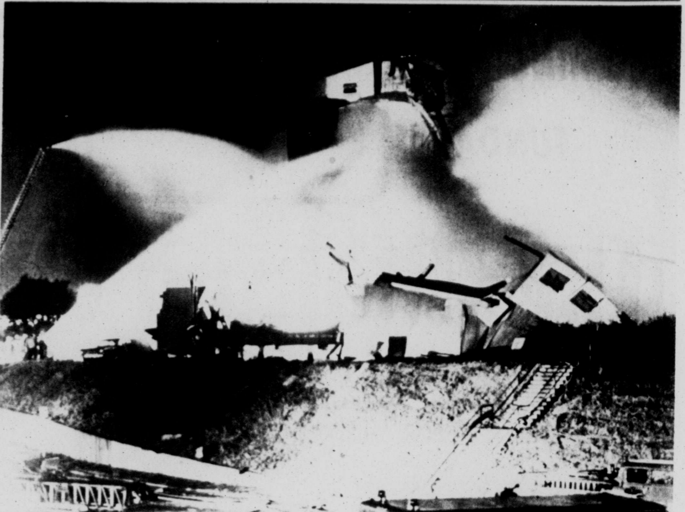
Firefighters doused the ruins of the Hiawatha Grain Co. elevator early Thursday following an explosion and fire. Two truck drivers and three
