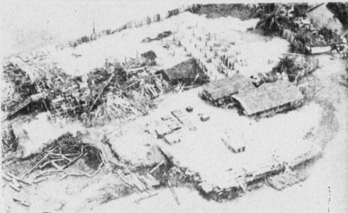
Some of the houses destroyed by an earthquake and a resulting 10-foot-high tidal wave Wednesday look like piles of sticks in this aerial view of a part of Guapi
