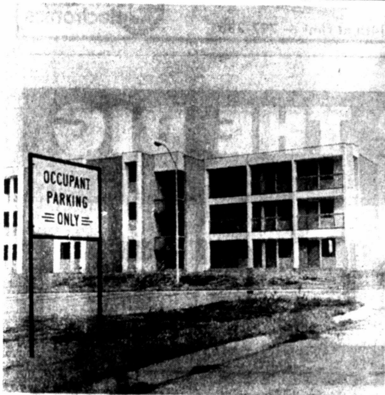
WEBB BECOMES PRISON HOME — Shown in the left panel is a dormitory formerly occupied by student pilots at Webb Air Force Base, but now the new home of minimum security federal prisoners. One of the exceptions is that the parking lot sign does not qualify the prisoners who will occupy the no-walls facility to bring along their cars. However, special privileges are given the inmates to qualify to serve
