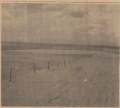
SITE 6, LOCATED ON THE JOE BROOKS FARM, shown above, filled to this level before the drawdown tube functioned. Another 8 feet of floodwater could have been stored below the emergncy spillway.
