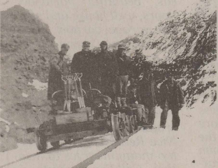
Section Crew on Cap - 1930's
