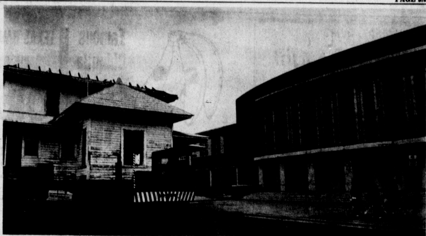
The past gives in to the future, as the Hill House is moved to make room for expansion of Midland High School.
