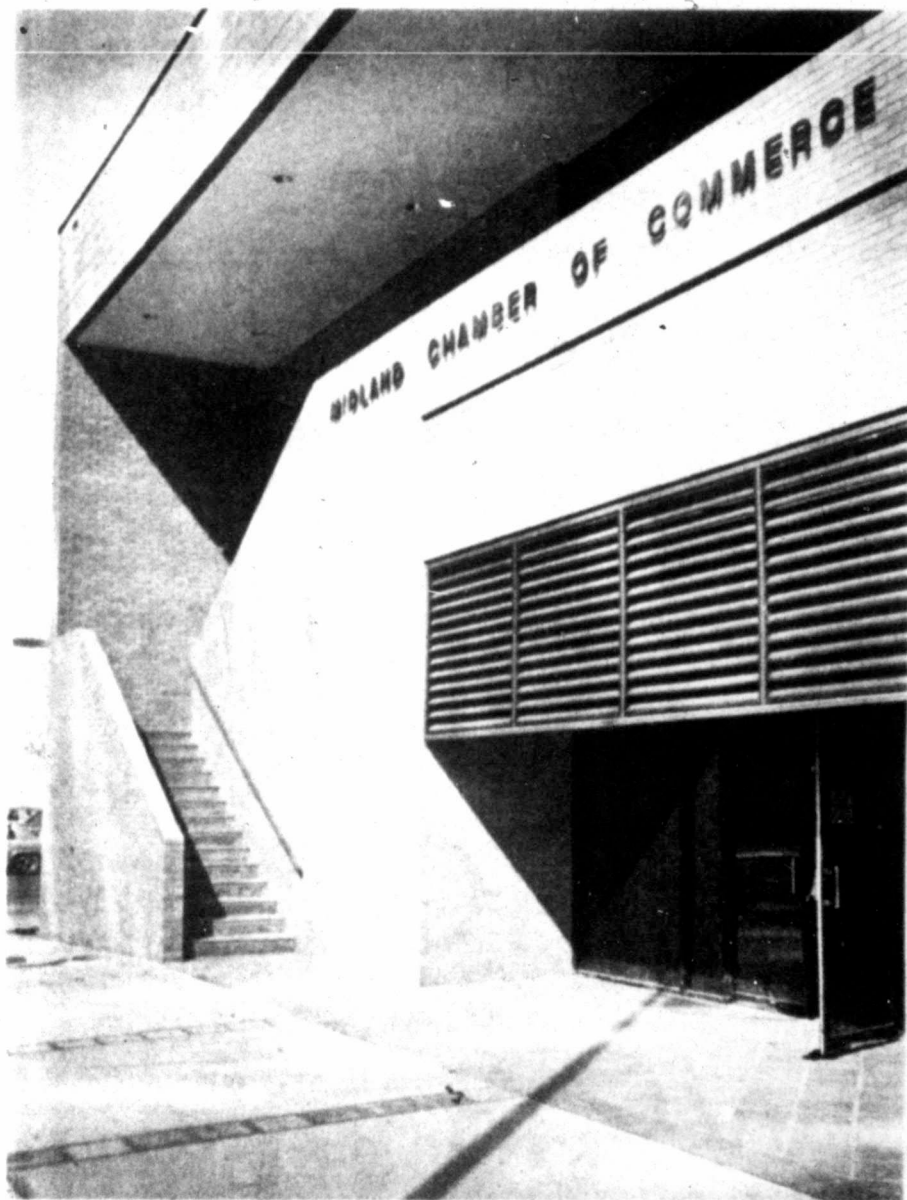
Overhanging ledges on the new Chamber of Commerce building were added for a purpose—to cut the amount of direct sun shining into the offices and thus saving energy to cool the structure. (Staff Photos by Brian Hendershot)
