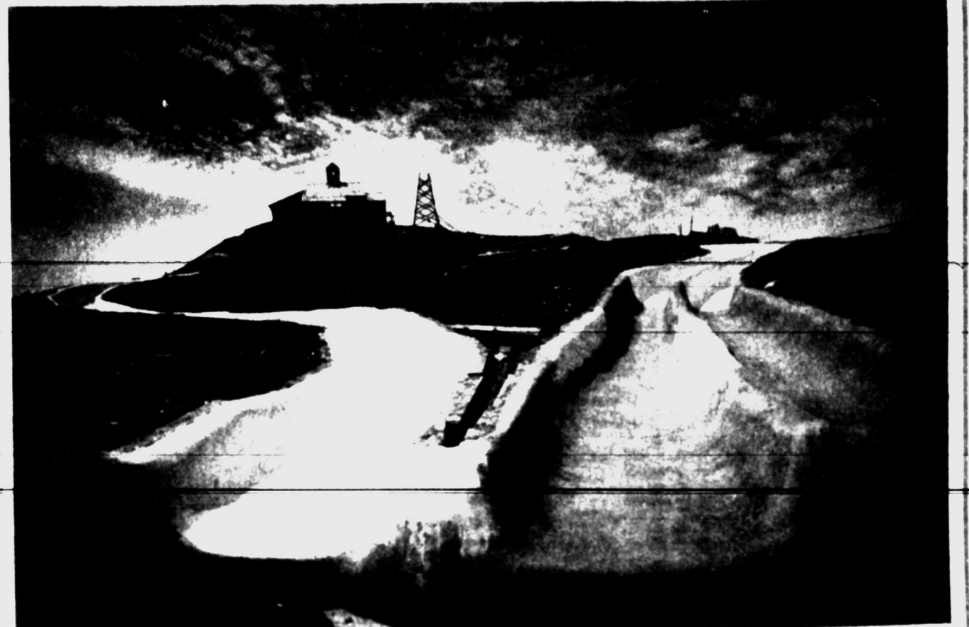
Curving down and around a manmade hill, concrete flumes are almost ready for the water to flow. This Mine Mountain River Ride will be one of the attractions of Wild River Canyon when the family fun park opens early this summer. (Staff Photo by Brian Hendershot)
