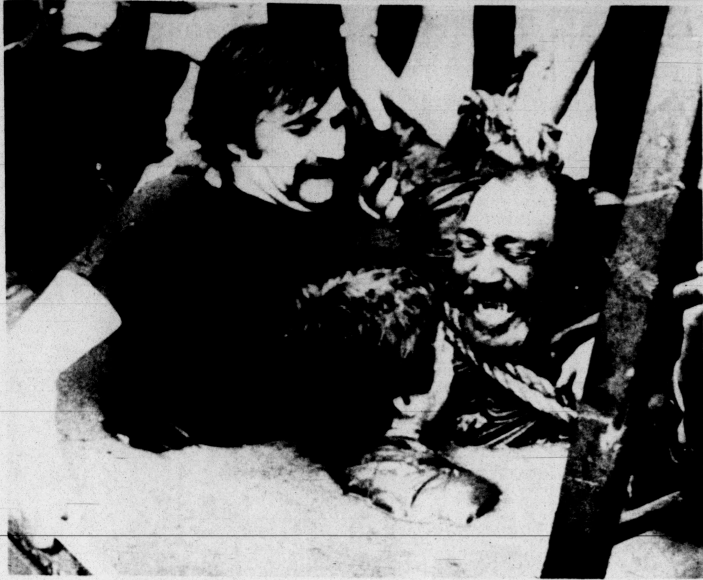
Myron Tucker, a 54-year-old city worker in Syracuse, N.Y., had a close call Tuesday when the six foot ditch he was working in collapsed and filled
