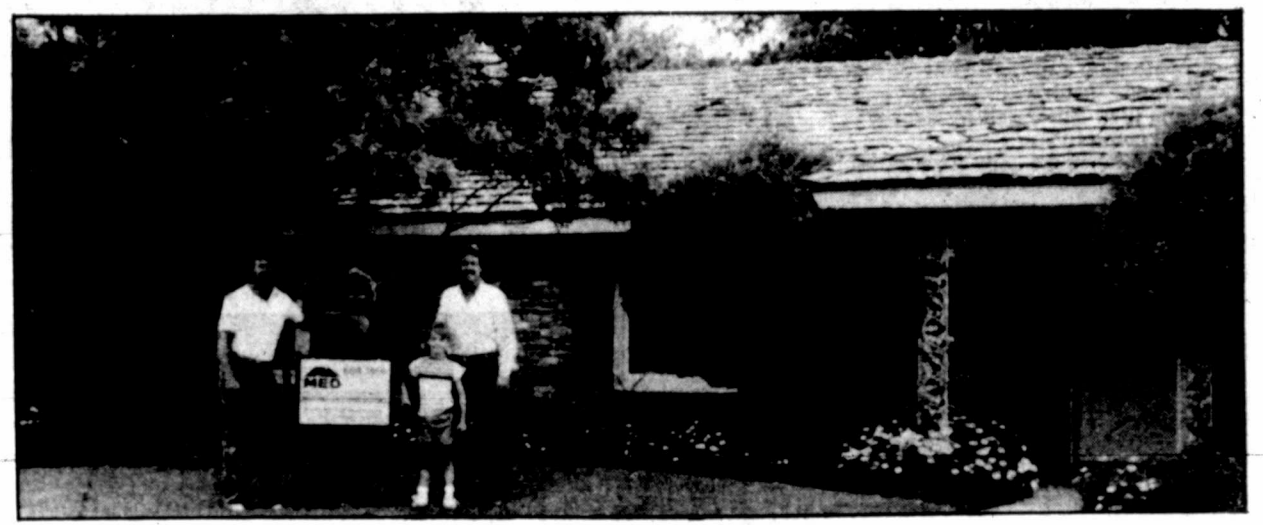
Gary Mitchell, Ellen Roberts, Midland Exterior Designs Owner Steve Tillman, and their number one playhouse estimator Reagan Tillman stand in front of Hugh and Jessie Gilmour's home on N. "L." This local company recently installed vinyl windows and maintenance-free soffit and fascia on this nice home. Be sure to watch for Midland Exterior Designs signs which indicate quality work is being done.
