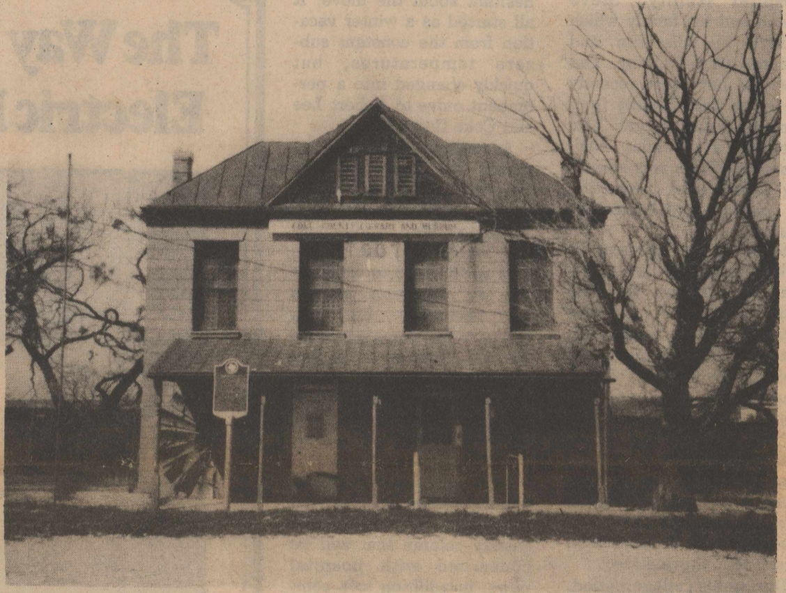
THE OLD COKE County Jail is the present-day Coke County Museum and is being restored by the Historical Commission and other interested persons. Located one block west of Highway 128 on Chadbourne in Robert Lee, the building has many historical items on display. Of great interest is the "hanging room" where outlaws were "put to death by hanging in the olden days".
