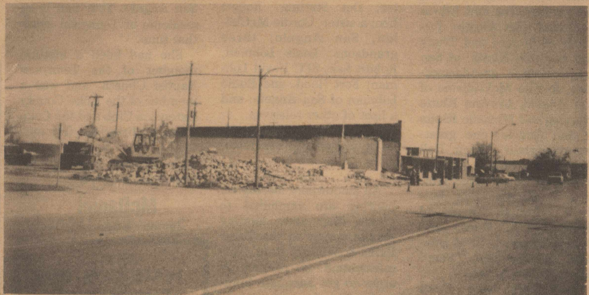
DOWNTOWN BRONTE WILL take on a new face-lift with the construction of a New Grocery Store. Construction began this week.
