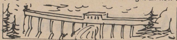
During the construction of the Hoover Dam, concrete had to be poured continually for two years.
