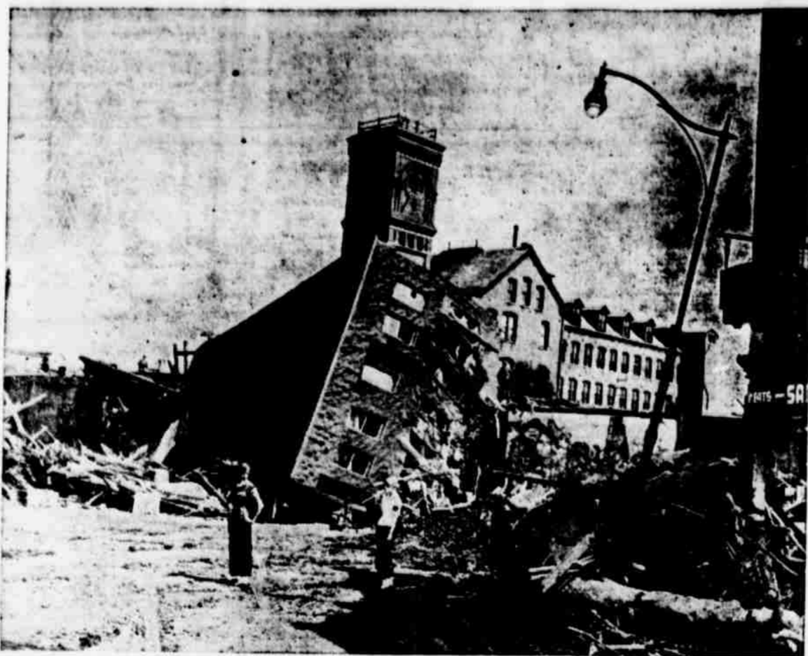
CRUSHED AND BROKEN, this 16-family apartment house in Waterbury, Conn., was left high and dry after the rampaging Naugatuck River receded. This was a sample of devastation in the flood which, according to the Red Cross, destroyed 1,328 houses and badly damaged 4,808. (Wide World Photo)
