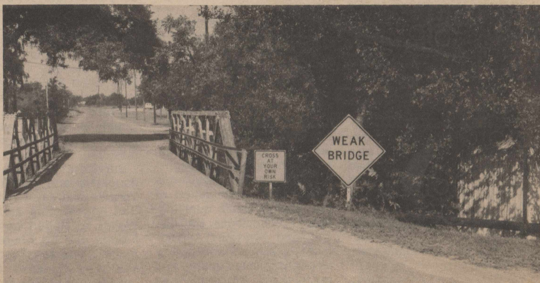
Completion for the new park road bridge in Bronte is expected in late Spring 1993. Motorists should exert caution when travelling in the golf course and park areas.
