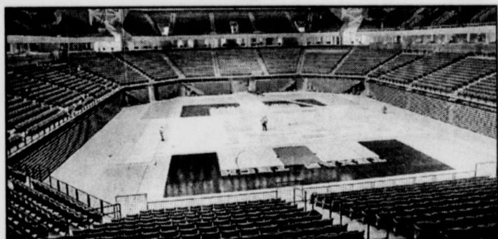
Construction crews are putting the finishing touches on the United Spirit Arena, Tech's $62 million complex.
