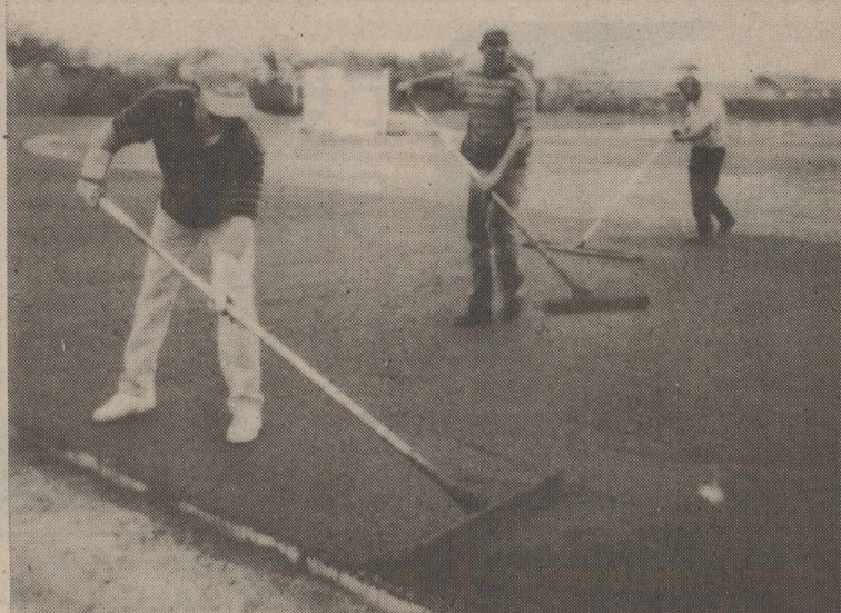
The new track facilities at Bronte ISD are nearly completed. The surface is complete except for striping.
