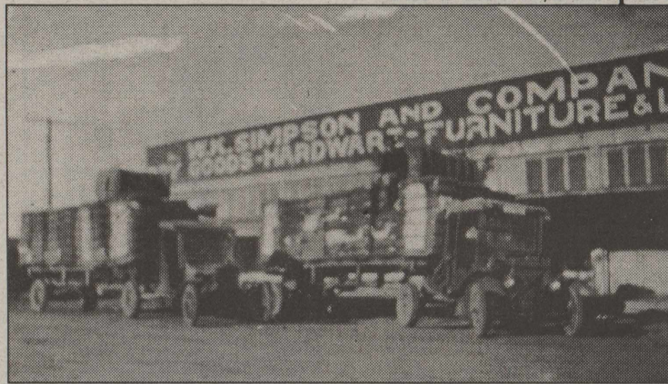
Simpson's business was located on Austin Street in the building now housing C & H Auto Parts and Hardware
