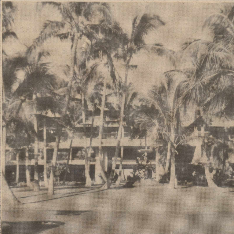
This is "ROCKFELLER's Hotel at Mauna Kea Beach.
