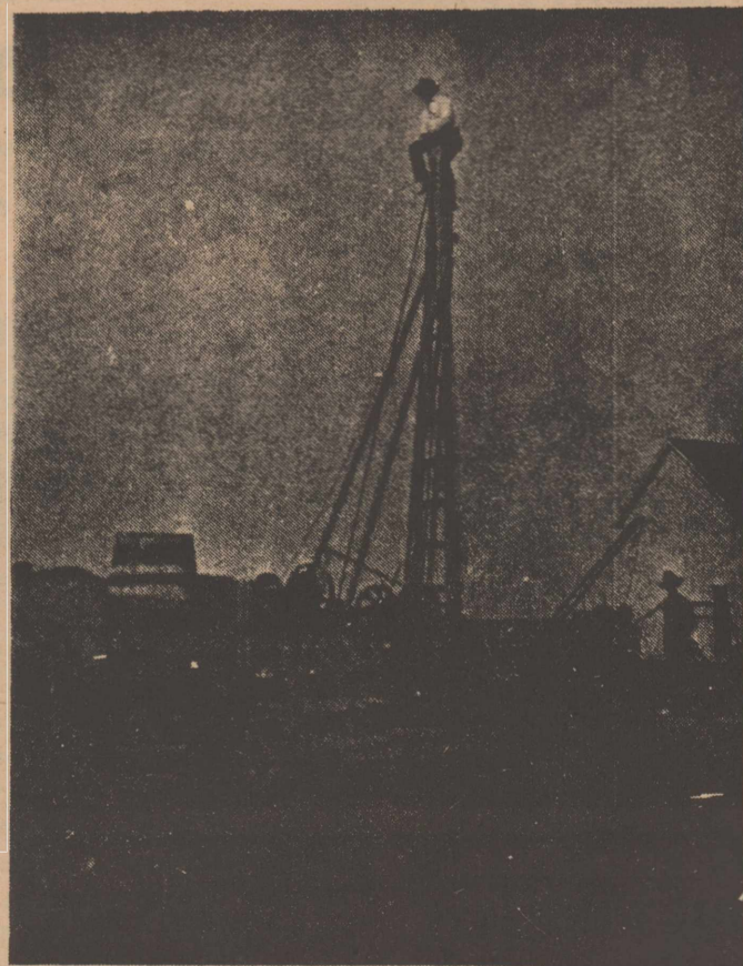
JIM MYLES IS SHOWN ATOP A DRILLING RIG, PROBABLY BEHIND THE OLD SAM MALONE HOUSE THAT WAS MOVED LAST WEEK.
