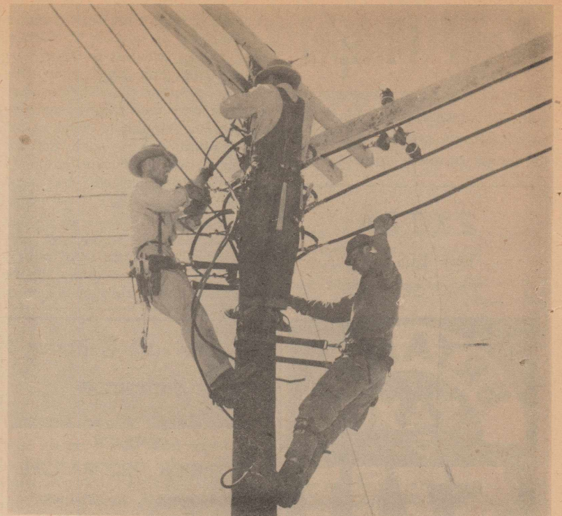
BOB LOMAX, ED CURRY, and PEC J. C. Wilson of Cabot, Arkansas, make final connections in the lighting system for the Reese softball diamond that is expected to open this week for night softball games. The area, located across from the hospital, will be lighted by 60 floodlights arranged in banks around the diamond.
