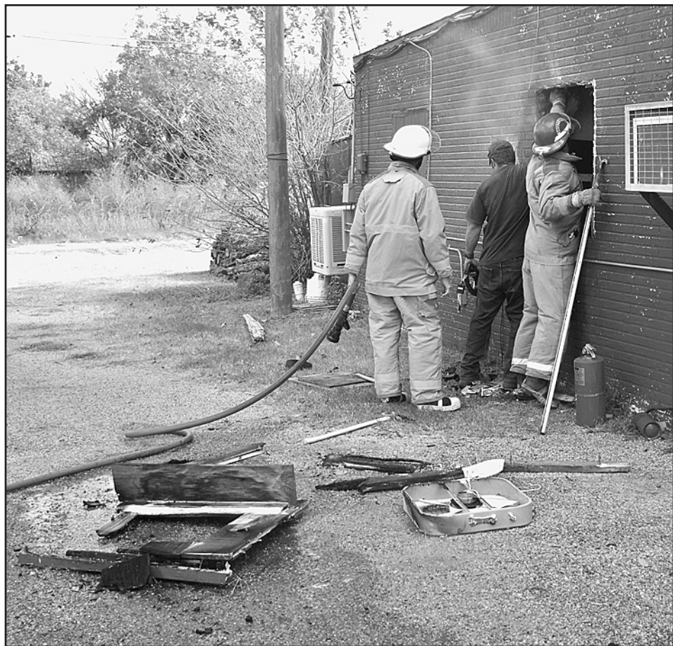
RESTAURANT FIRE —The Haskell Volunteer Fire Department responded to a fire at the Pit & Grill Thursday afternoon, Nov. 11 at about 2 p.m. The call was placed by employees at the neighboring Sonic who reported smoke coming from the area of an exhaust fan. Owners Shelly and D.L. Cooper had just closed and left the restaurant after the lunch run. Quick action by the owners, who had a fire extinguisher; a bystander, Greg Hearn, who pulled the fan from the building; responding Fire Chief Randy Shaw with a fire extinguisher on board the Haskell County Fire pickup; and the responding fire apparatus unit and firemen, limited the damage from the blaze to the frame around the fan. The inside of the restaurant sustained some smoke damage and water damage, but the restaurant reopened Friday for the regular meal service.
