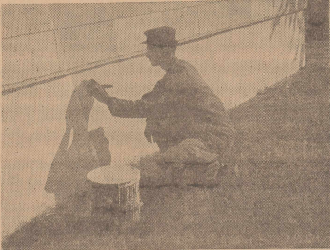
PAINT PRESERVED —A/B Harry Slater applies paint to the base library fountain as a major phase of the Preventive Maintenance program. Interiors and exteriors of buildings are painted.
