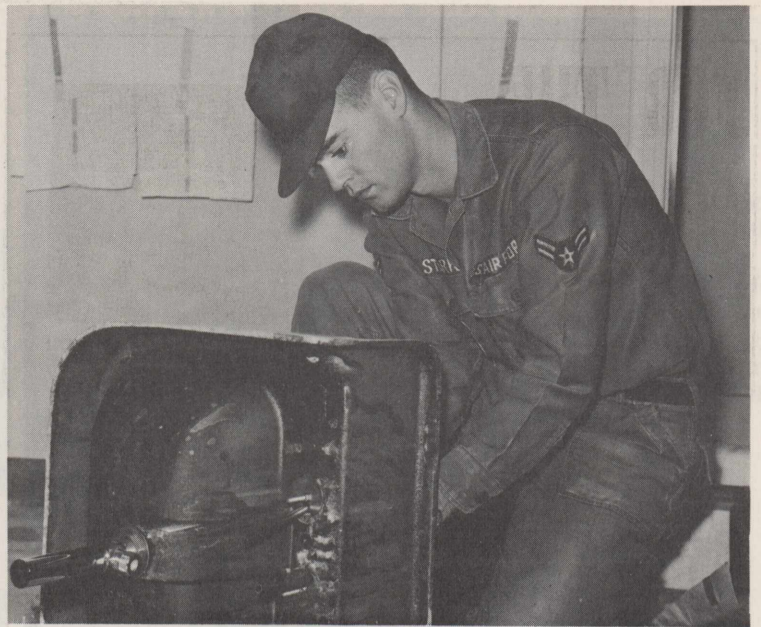
HARD AT WORK —A1C Robert C. Stark, December's Airman of the Month, plumbing specialist assigned to Civil Engineering Division, replaces seals and gaskets while installing new fixtures in airmen's quarters. (USAF PHOTO)
