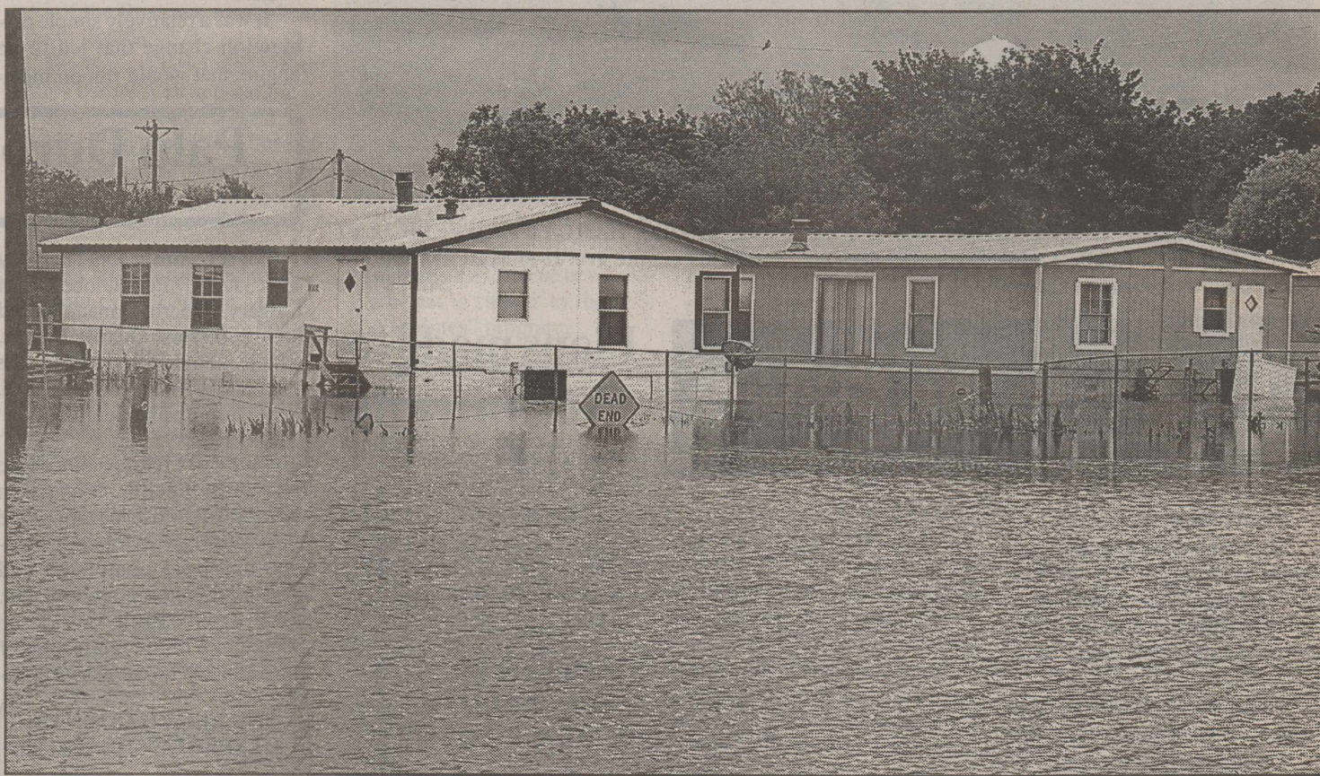
CONTINUAL RAINS HAVE FLOODED THE AREA BEHIND ACE HARDWARE, ON THE SOUTH SIDE OF HWY. 62
