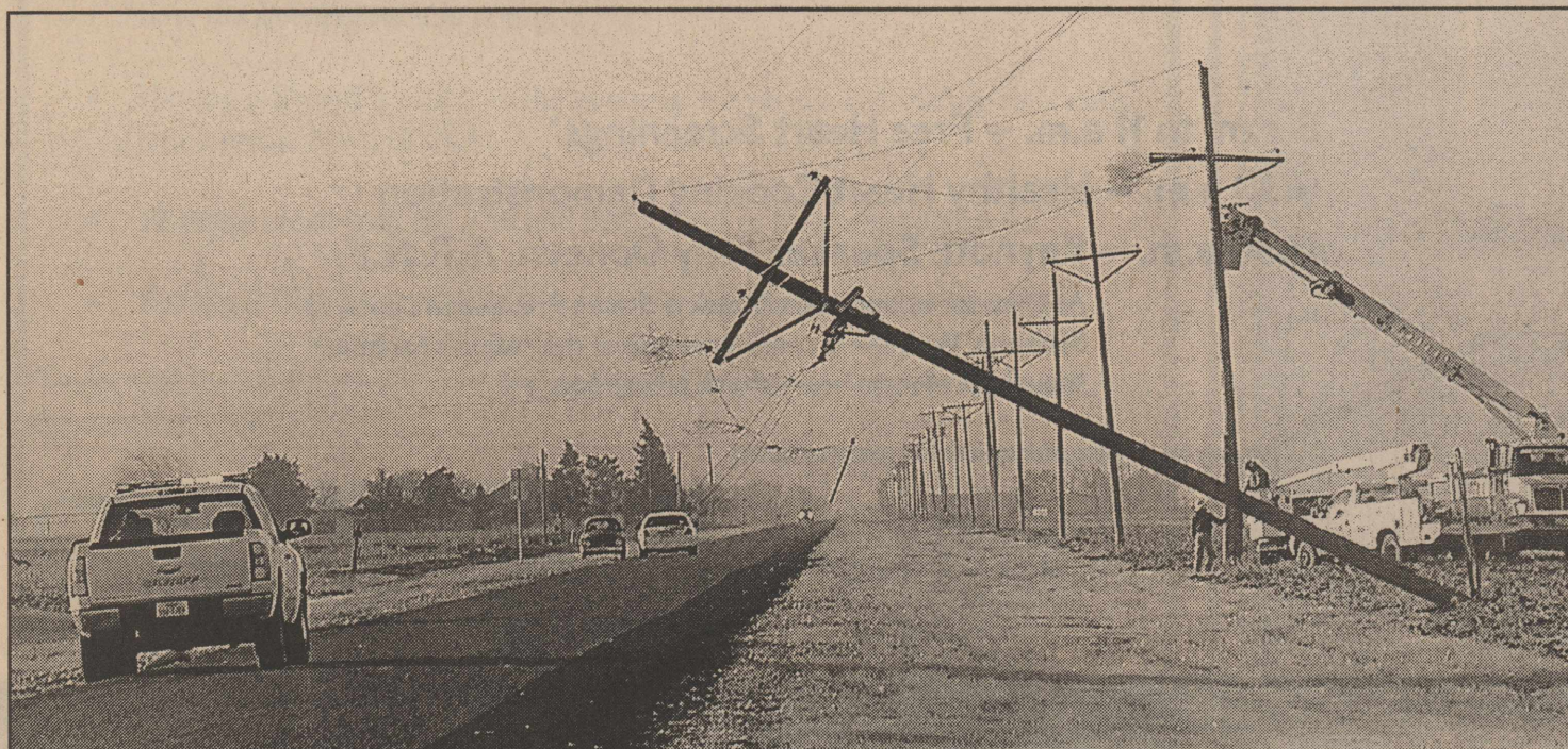
HIGH WINDS DOWNED POWER LINES in the Aiken area on Hwy. 2301, the morning of January 29. Peak gusts were registered at 59 mph at 5:20 a.m. Staff Photo
